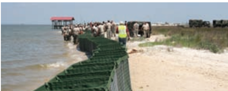
Dauphin Island: the four-mile double-walled structure consists of baskets (supplied by Hesco-USA) which are staked into the ground, and which are filled with sand and a special powder-like blend of polymers that react with oil and within minutes turns it into a solid, rubber-like mass. The solidified hydrocarbons can be swapped with fresh polymers as and when necessary, and the solids taken away for non-hazardous disposal, or even recycling into products such as asphalt.
