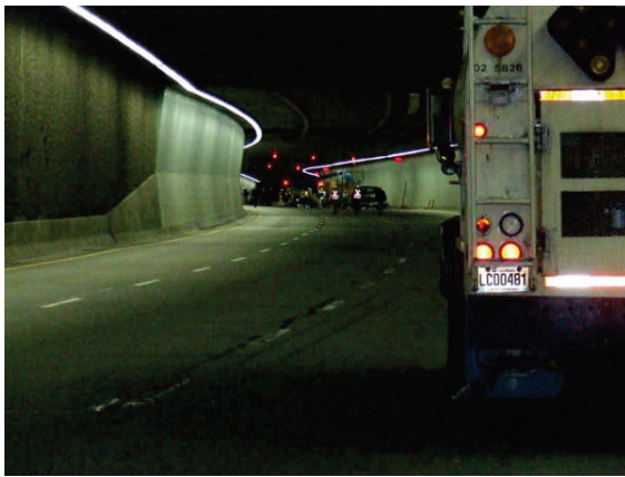
Figure 2. AlarmEye VID system working in a road tunnel
